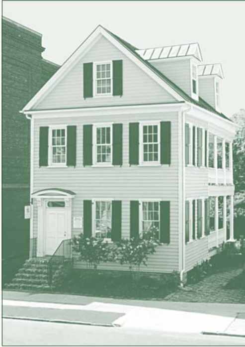
113 Calhoun Street: A Center for Sustainable Living
